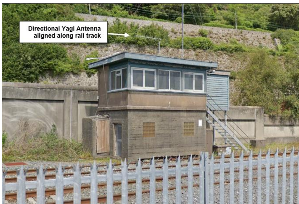
Figure 2. Example of Analogue Train Radio installation using a Yagi Directional Antenna
